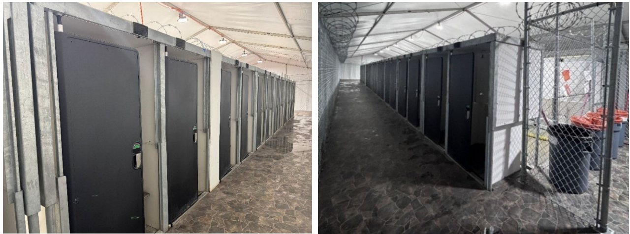
Figures 19 and 20. Shower Facilities; Observed January 21, 2026
